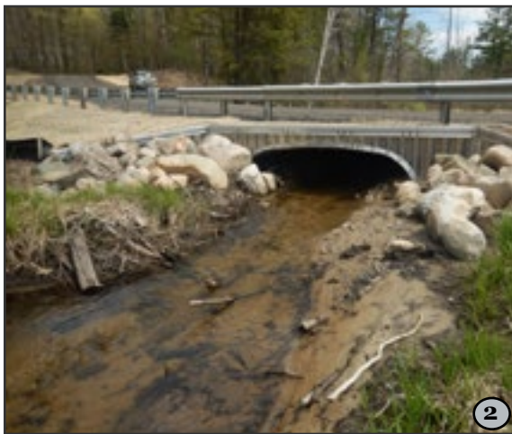
2. Oversized culverts with metal grated tops and soil bottoms let more light in and create conditions that are more natural and easier for amphibians and reptiles to navigate.
