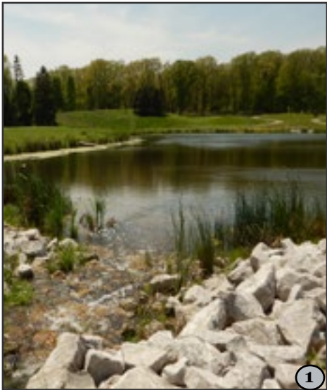
1. Stormwater management can be designed to provide flood retention, water filtration, and habitat value. Sites Like Groesbeck Drain serve these functions.
