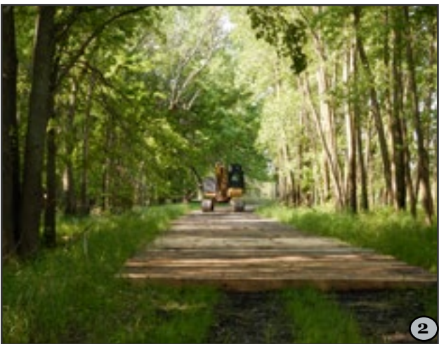
2. Construction mats help to reduce the compaction of hydric soils and prevent ruts caused by equipment.
