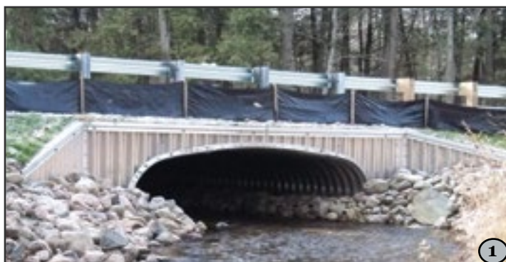
1. This open-bottom arch culvert allows species like the Wood Turtle to follow stream corridors safely while reducing the risk of road mortality. For an additional illustration of this structure, see Figure 15 in development techniques.
