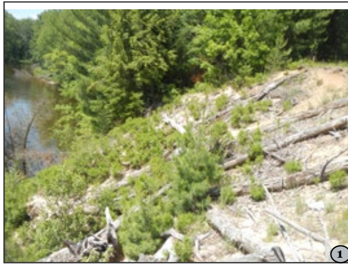
1. Placement of logs along the banks of a exposed river bank helps stabilize soils while still allowing for movement of turtles to find nesting areas.
